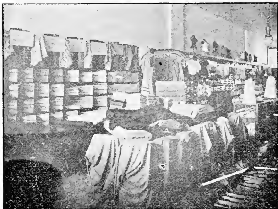
INTERIOR VIEW OF STORE
